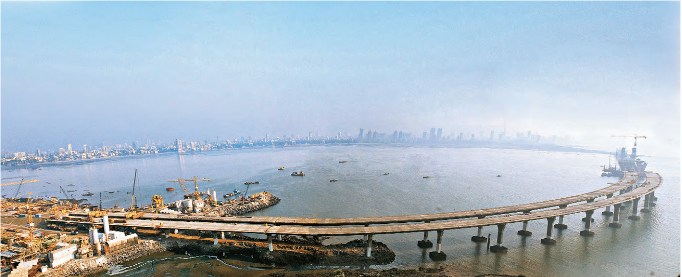
When completed in 2008, the $ 300 million, 5.6 km long Bandra Worli Sea Link in Mumbai will save the city's commuters $ 22 million every year
